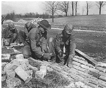
CCC Workers Constructing Road
